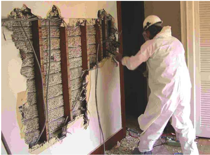
Fig 2 – Old Armored Cable Being Removed From House IL-1
